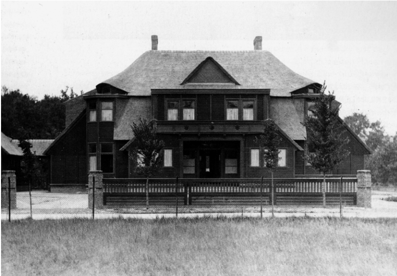
(FIG. 26) — Henry van de Velde's home, De Tent , in Wassenaar, The Hague (1920-1921). Prefabricated construction in wood from the Silesian firm Christoph & Unmack, based on a model adapted by van de Velde.
